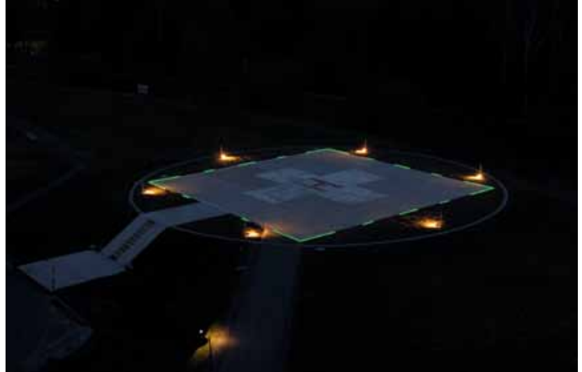
Figs. 2 and 3: This innovative LED strip-based ground lighting system is now to be employed for the first time (Photographs: T. Wysk)
